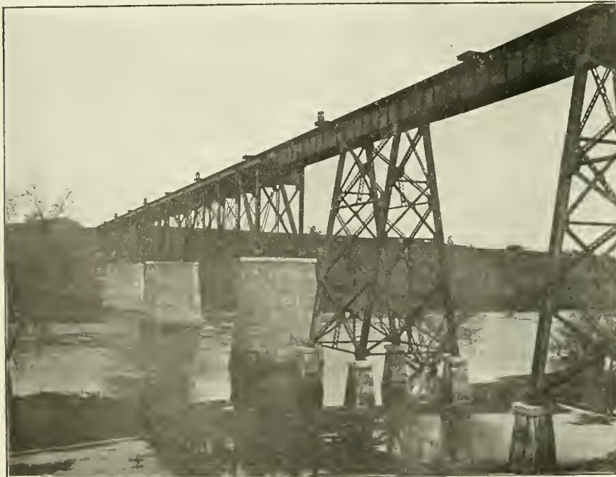
BRIDGE AT WATERFORD ON THE SOUTHERN PACIFIC.
